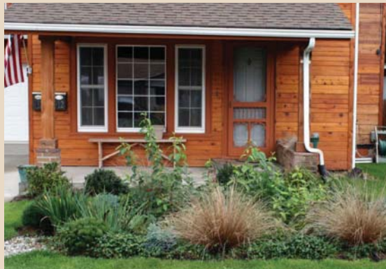
Rain garden installed and photographed by Stewardship Partners.
