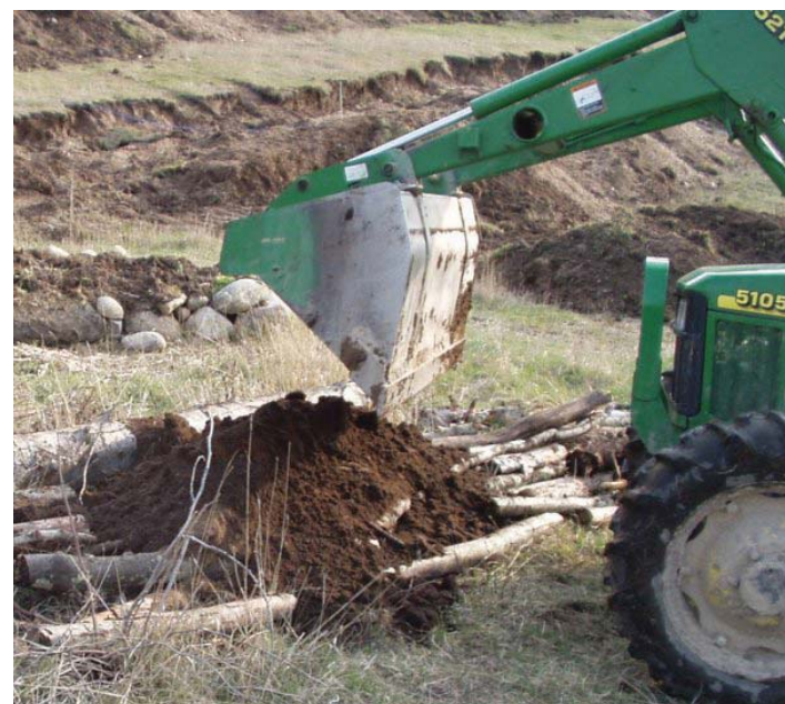
5. The first of many loads of soil and compost are added.
