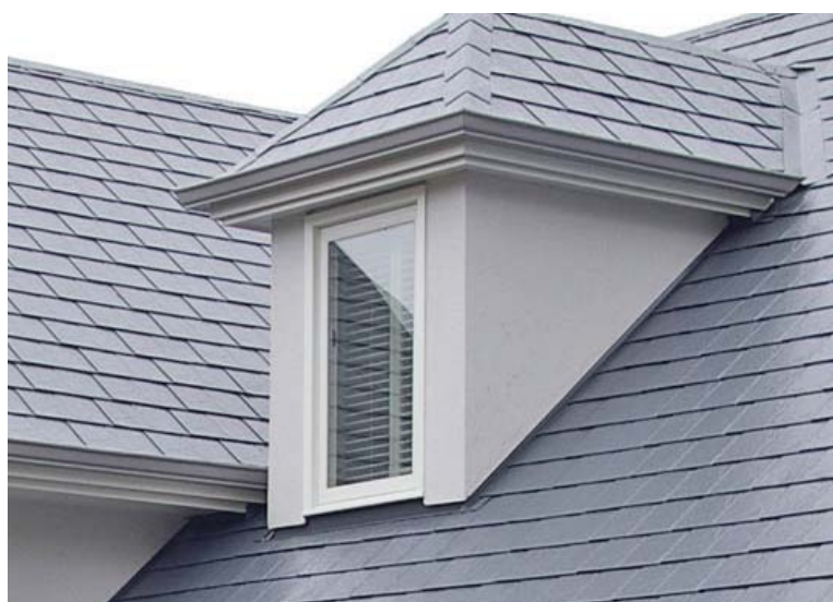
A Firewise roof using slate roofing materials.
