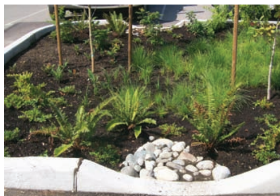
Rain garden at the Evergreen State Fairgrounds.
