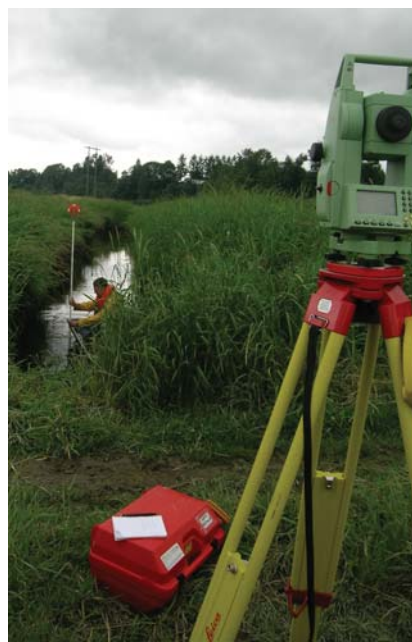
Conservation District Engineer Ryan Bartelheimer surveys the slough prior to construction.
