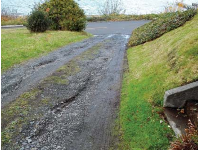
Alan's driveway before.
