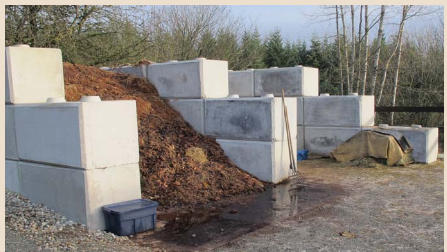
New manure storage bins funded by Clean Water District fees.
