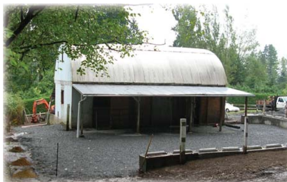
Now mud-free after a gravel pad was installed and drainage added.
