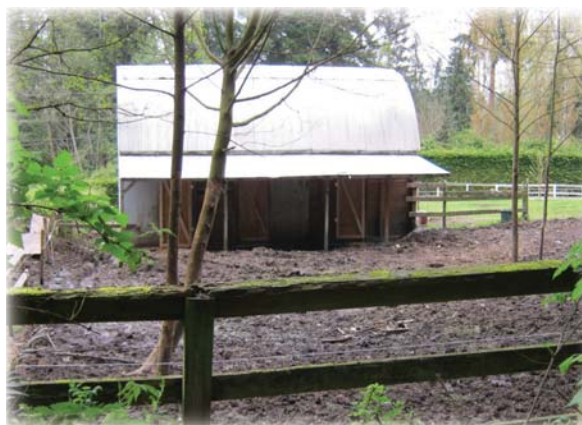
The photo above shows a muddy slope leading down into this barn.
