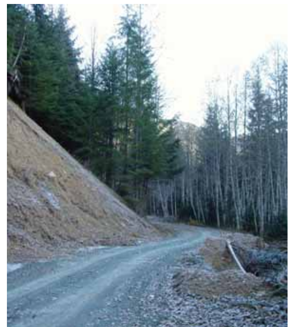
A typical steep hillside found on upper watershed roads that contributes to sediment downstream.
