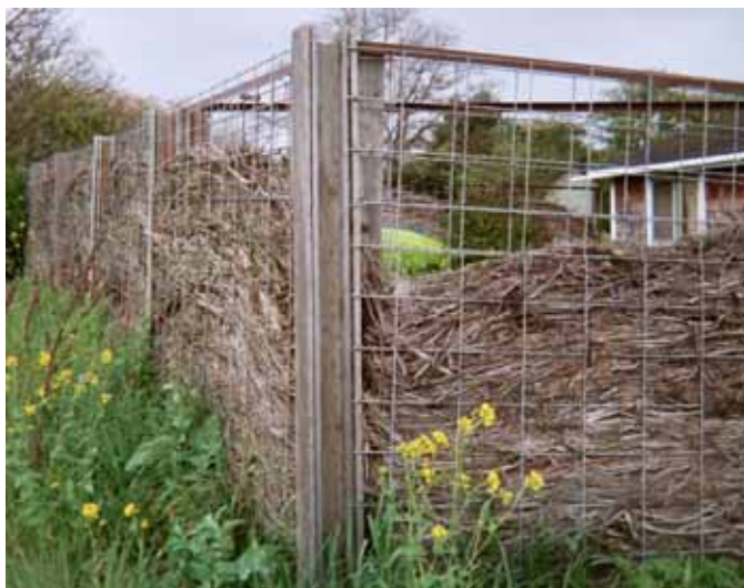
Compost Fence on Whidbey Island
