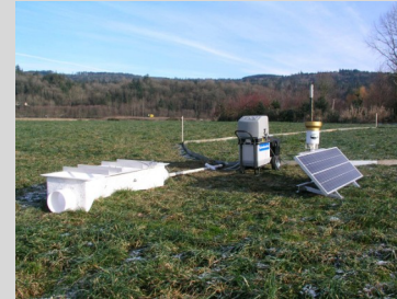
WSU Research plot monitoring equipment installed and field-proved by SCD personnel.
