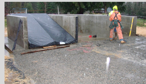
SCD District Engineer Paul Smidansky puts the final touches on waste storage bins to help manage manure at a local farm.
